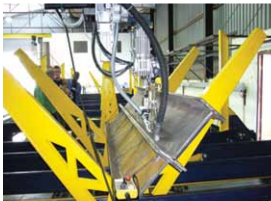
The first ever flip-flop table to manipulate girders for welding.
