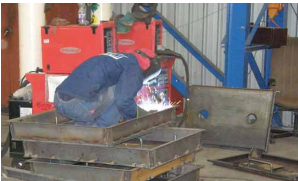
GMAW, using Fronius welding machines with Argoshield 5 gas and Bohler EMK 6 solid welding wire is used for almost all of the welding at AGS Engineering.
