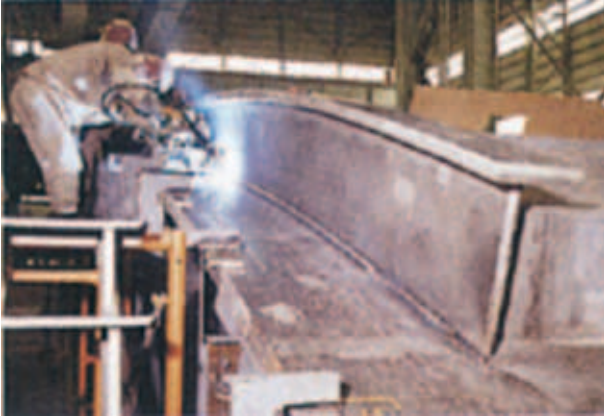
Figure 3: Automatic high-current GMAW of spherical aluminium LNG containers [4].
