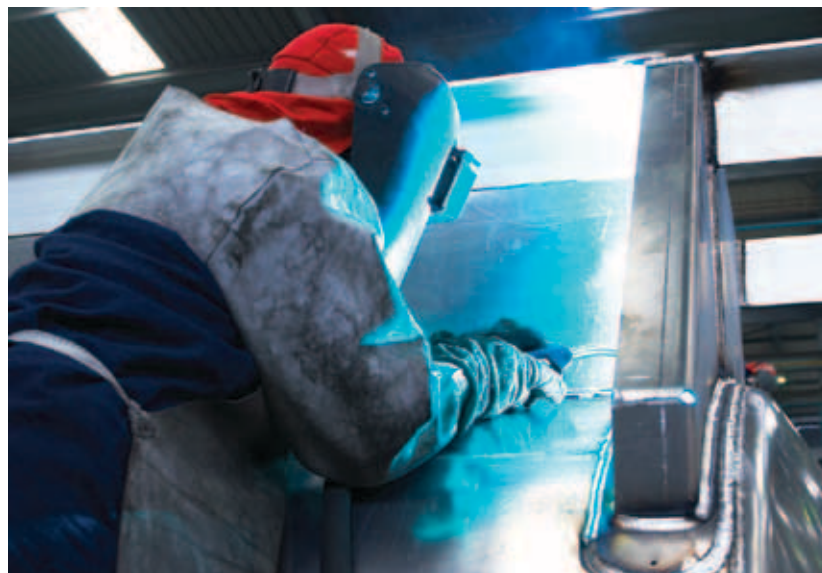
Fuel tankers are all fabricated from welded aluminium.
