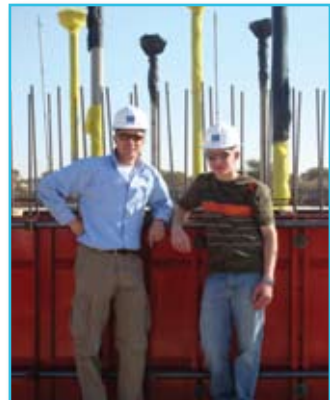
Wian Steynberg (left) from Kwezi V3 Engineers, Kimberley, took Gideon van Tonder – a matric student from Diamantveld High School in Kimberley who has shown interest in studying civil engineering – on a site visit to Kathu.
