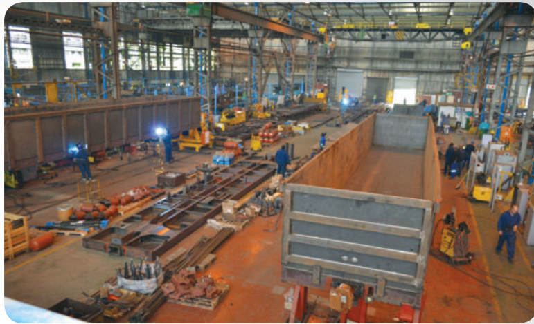
Transnet Rail Engineering's Bloemfontein facility is currently the lead fabricator for South Africa's freight wagon fleet. According to Brian Molefe, Transnet group CE, Transnet's latest transaction would create and sustain 30 000 local jobs and contribute over R90-billion to the economy.
