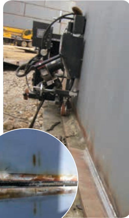
Above: A Lincoln LT7 tractor and Lincoln Flextec 650 power source is being used to complete the floor-to-shell outside circumferential weld using the submerged arc process. The same equipment is used to weld the tank base. Left: A completed AGW weld on a 20 mm bottom strake.
