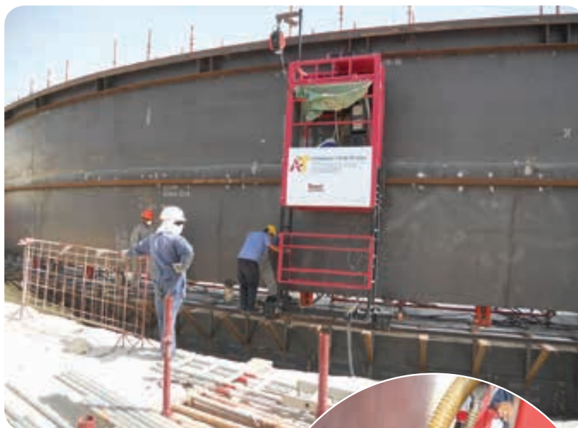
Above: The 'jack-up' method, or the 'top-down' construction method has some access advantages, because all the welding work is done closer to the ground. "By keeping the bulk of the work at a height of 2.4 m, access is much easier," says Bronkhorst.
