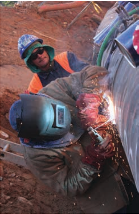
Above: Böhler Welding's combination method using cellulose-coated electrodes offers maximum security against cracks. The root is welded with BÖHLER FOX CEL and the other layers are welded with filler materials matched to the strength classes of the pipe material.
