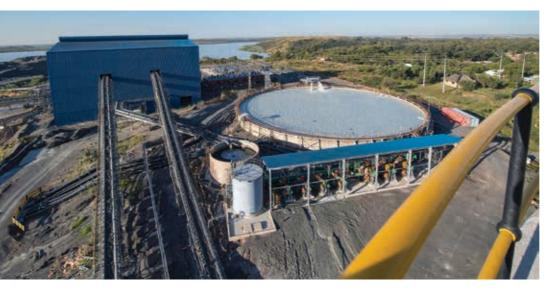
designed for a fresh feed rate of 375 t/h and a 152% circulating load.
