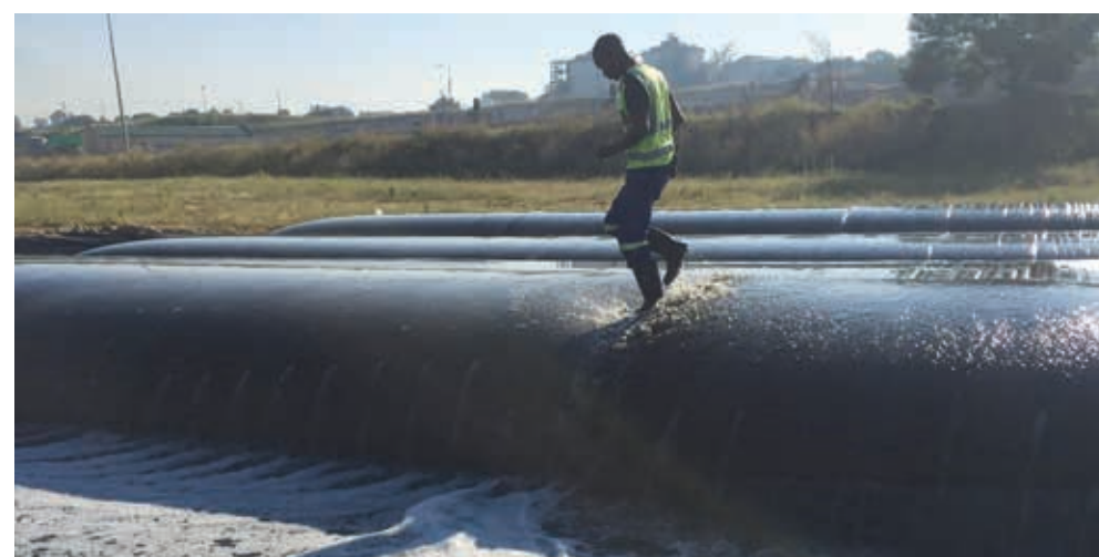
The benefits of using Fibertex geobags for sludge removal include ease of operation, efficient retention of solids, compliance with environmental regulations and cost optimisation – this dewatering system is passive and does not require constant monitoring and maintenance.
