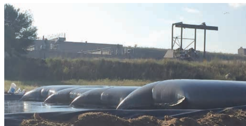
A recent local project where the Fibertex solution was used to remove sludge from the existing mine tailings facilities.
