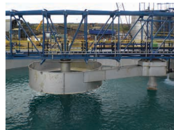
The thickener feed arrangement with P-Duc.
