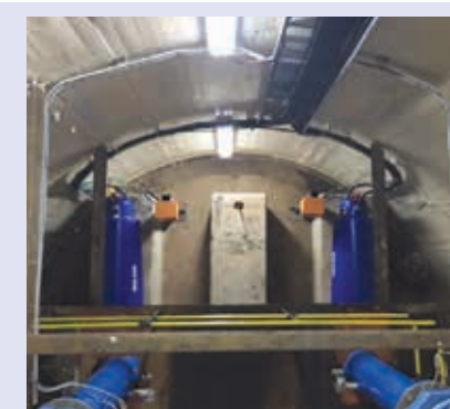
Sulzer XFP pumps (shown left) wait to pump 220 l of sewage every second (above).
