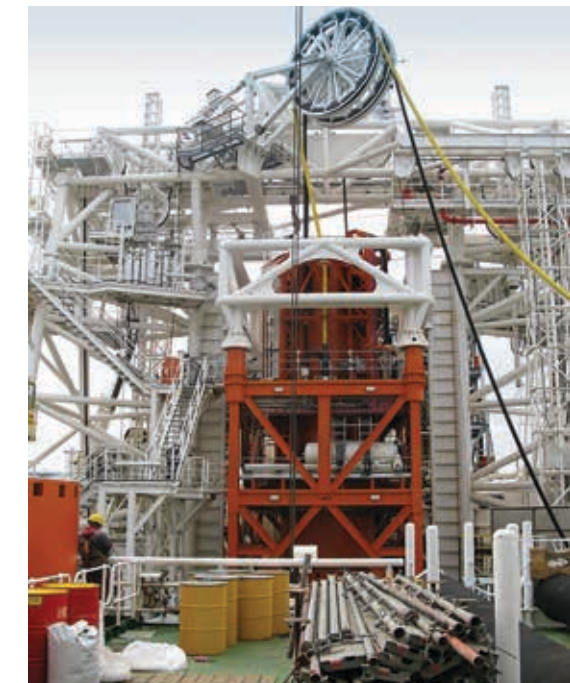
A front view of the launch and recovery system (LARS) and SBT during installation.
