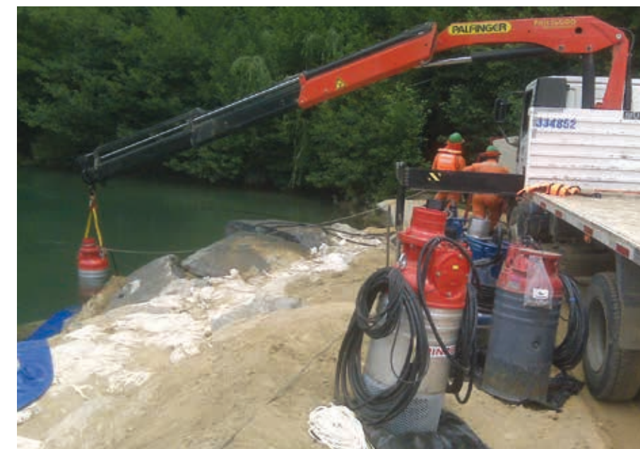
Grindex Maxi L pumps being used to check the depth of the clean water dam. IPR has Grindex dewatering pumps from 1.0 kW to 90 kW and Grindex sludge pumps from 2.0 to 10 kW available for rental.
