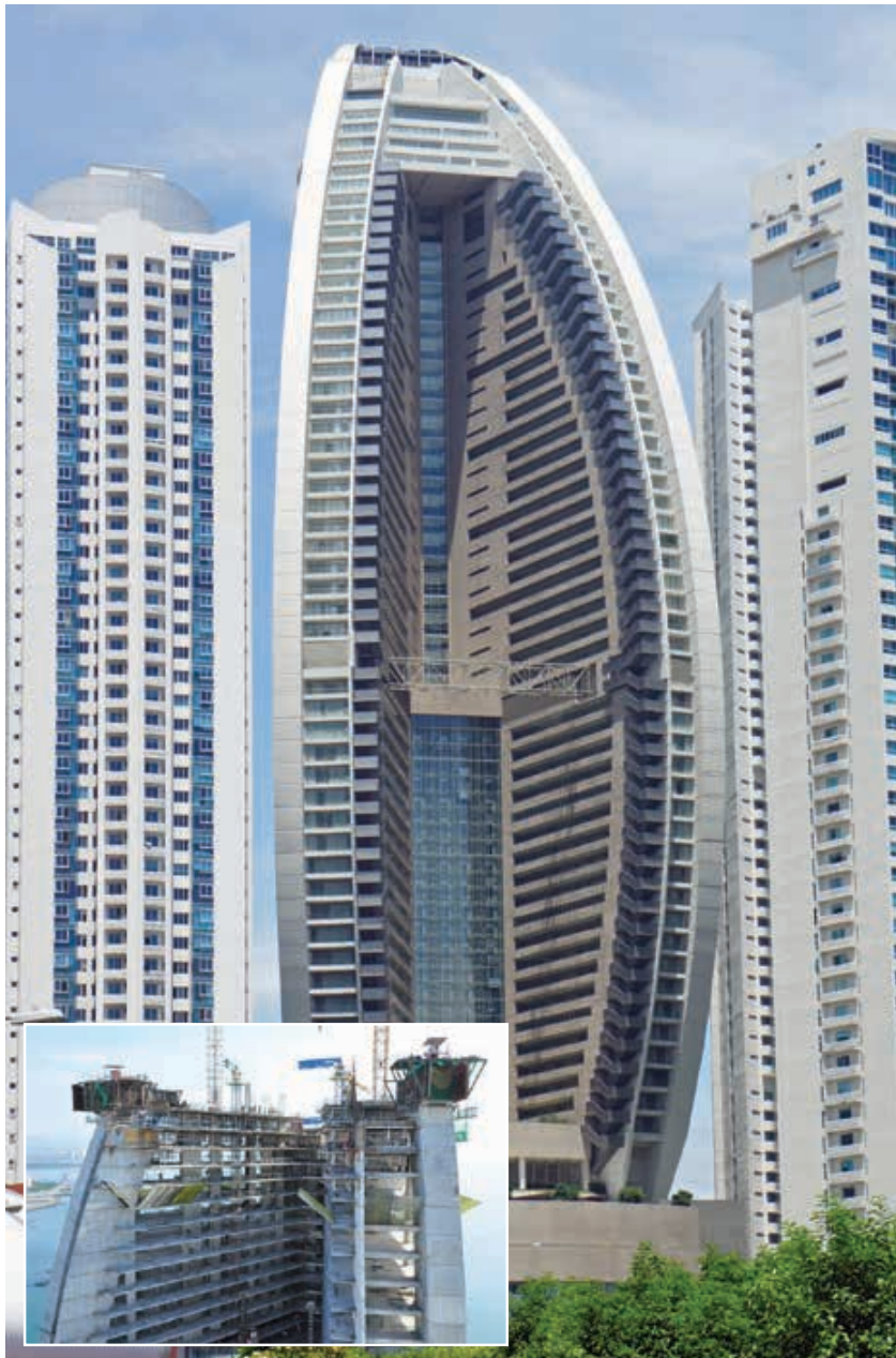
For the Trump Ocean Club Hotel and Casino in Panama City RBES designed and manufactured the hydraulic shutter-lifting systems for the lift shafts, mast and the hotel's arcs (inset), which were required to position the shuttering to form the parabolic shape.
