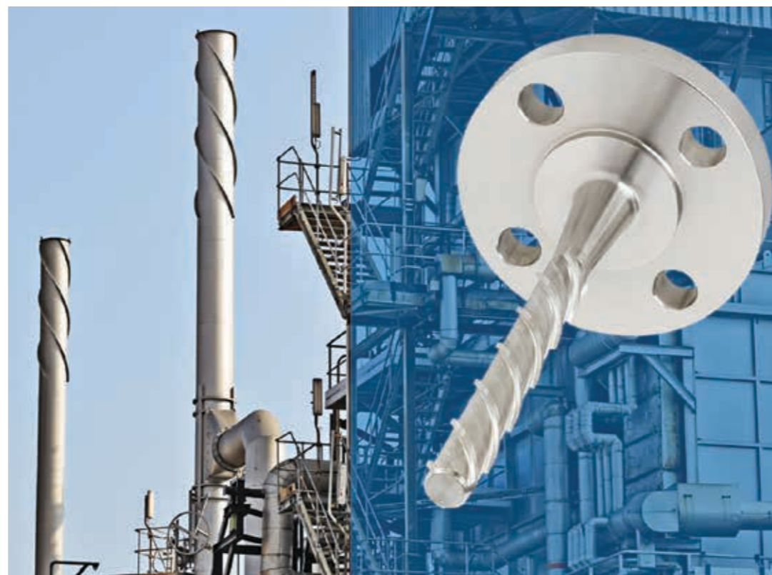
Industrial chimneys with a Scruton helix and (inset) a thermowell with a ScrutonWell® design. The helix diverts the wind or flow upwards on one side and downwards on the other, preventing the formation of vibration-causing vortices.
