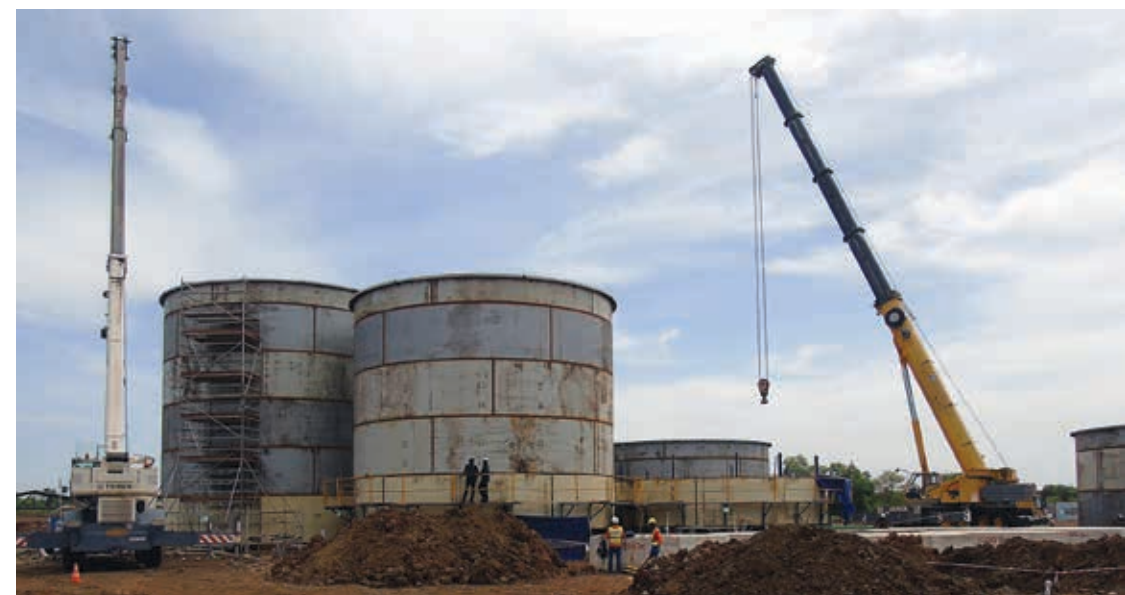
A recent view of leach tanks under construction at the Boungou site.
