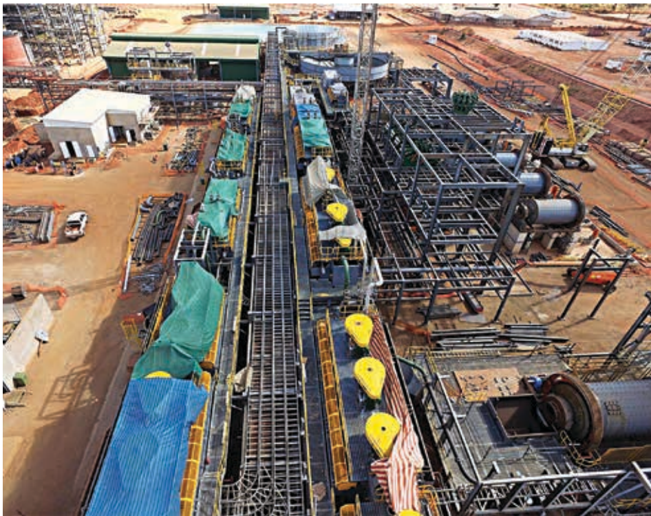
The flotation section of the Balama plant under construction (photo: Syrah Resources).
