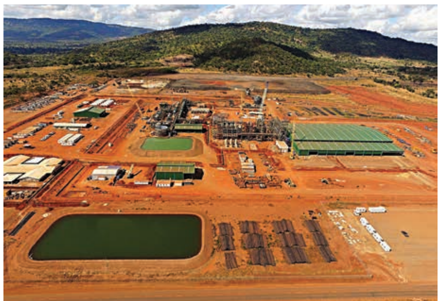
Looking south over the Balama site. This photo is from May this year (photo: Syrah Resources).
