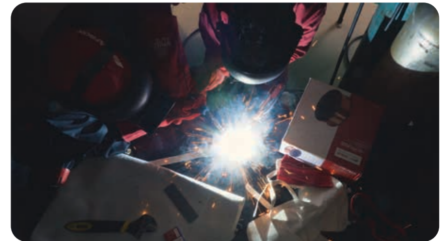
On completing their Trade Tests later this year, apprentice welders trained at the Academy may be among the first in South Africa to graduate from the new QCTO programme as Red Seal artisan welders.
