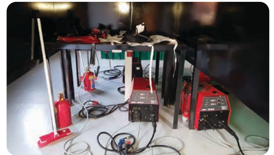
Built by coupling together a collection of second-hand shipping containers, welding booths were added and equipped with Afrox-sponsored multi-process welding equipment.
