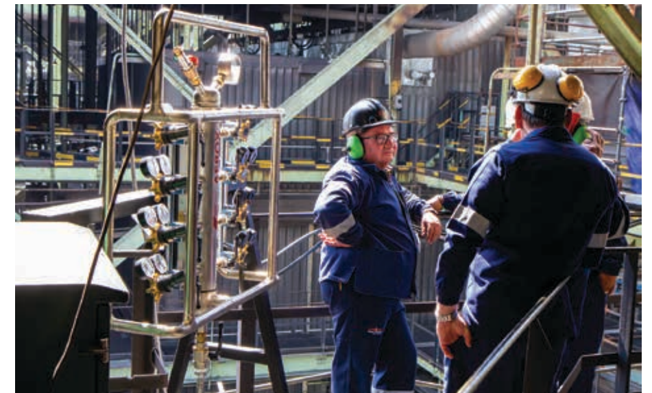
Afrox's MUPP solution leaves the gas cylinders on the ground in a safe, secure and convenient fenced off area. A single steel hose connects the gas to a pressure-regulated MUPP with eight connection points on each level of the boiler being repaired.
