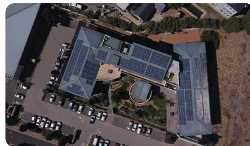
Lesedi has also recently completed the design and installation of a 142 kW solar electric installation for its head office in Century City, Cape Town.
