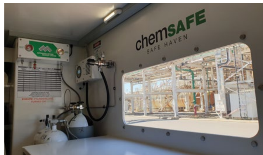
A ChemSAFE refuge chamber create a totally sealed environment with its own atmosphere.
