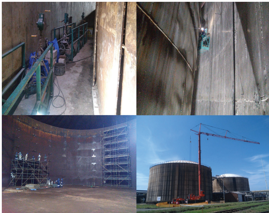
thyssenkrupp Uhde is inspecting & refurbishing a 20-year-old ammonia storage tank for increased lifespan and continuous safe operation.
