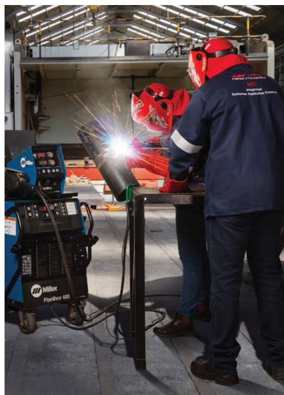
RMD eliminates the need for a hot pass, resulting in a process that often replaces the conventional GTAW process for welding large-bore pipes.
