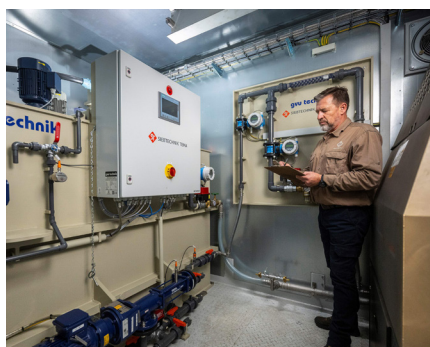
Left: The Multotec demonstration and decanter centrifuge comes in a 40-foot container with a small footprint.
