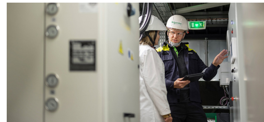
Schneider Electric's field services, proactive maintenance and asset management offerings offer opportunities for industrial plant to use automation, artificial intelligence (AI), and the Internet of Things (IoT) to upgrade and modernise their operations, helping them to remain competitive and sustainable.
