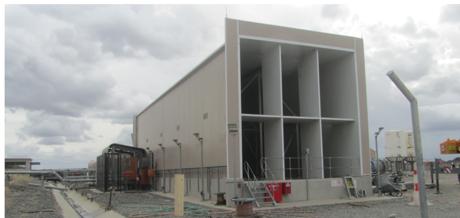
For the Venetia diamond mine, BBE designed and commissioned a new primary air-cooling (BAC) and ventilation system comprising two water-chilling refrigeration machines and multiple air coolers in August 2022.
