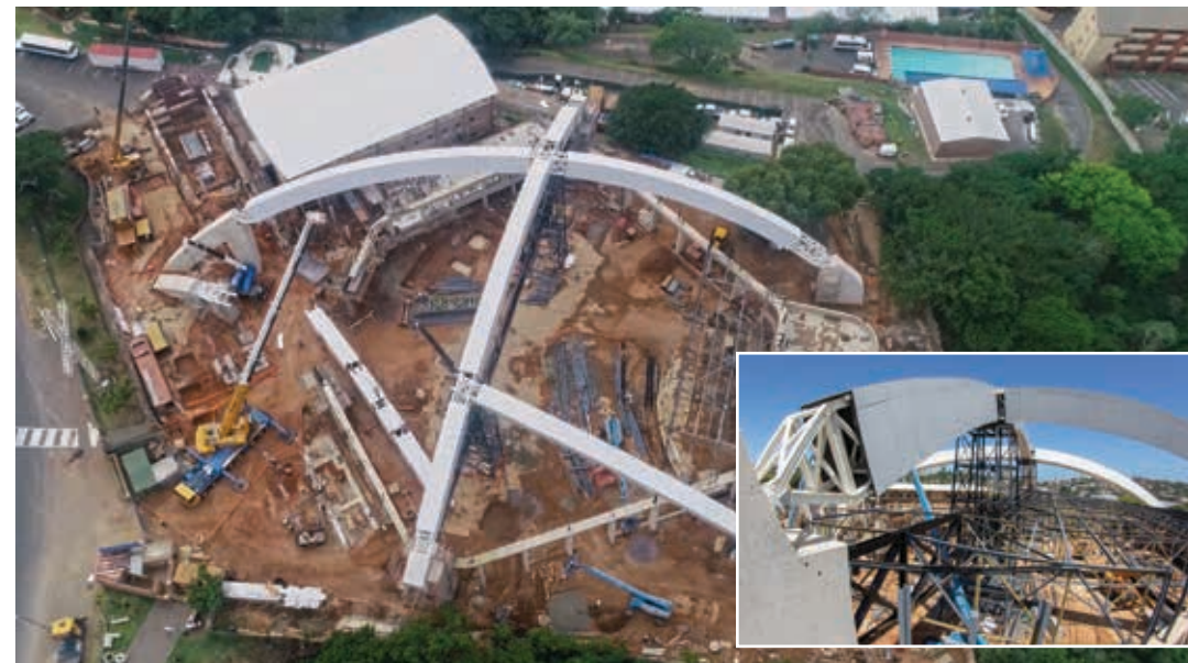
The innovative design of the Durban Christian Centre lay in the geometry of the large roof arches, inclined in different planes, which provide support for the roof as well overcoming tight site access issues. Inset: A view of the complex structural detail of the steelwork for the Durban Christian Centre's roof.
