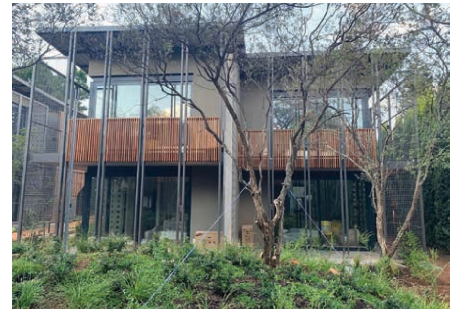
The steel mesh of the wraparound balconies of the Peech Hotel – winner in the ArcelorMittal South Africa Architectural category – was used to create the articulate façades of an urban village, while also serving to integrate the building with its green surroundings.
