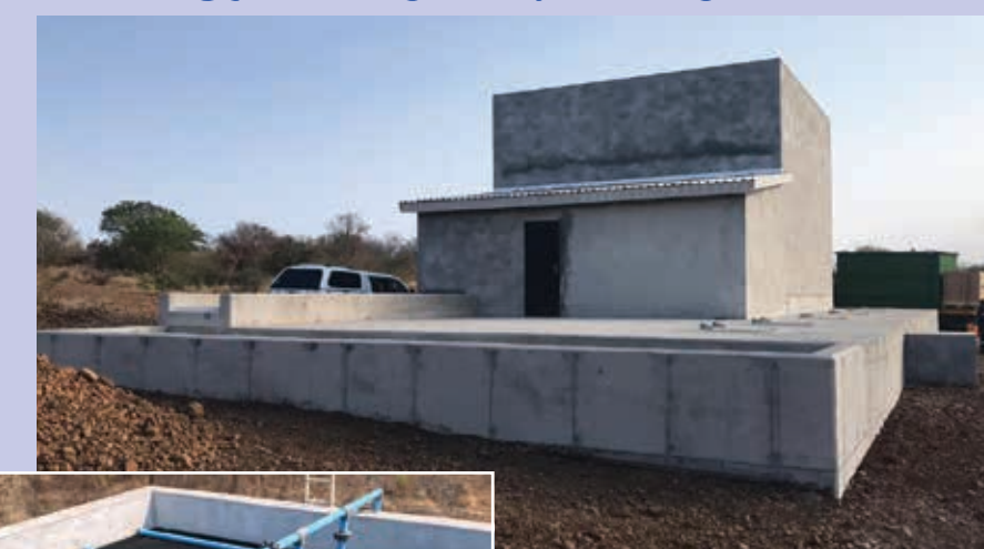
Above: Veolia's 400 m³/day civil-based sewage treatment plant.
