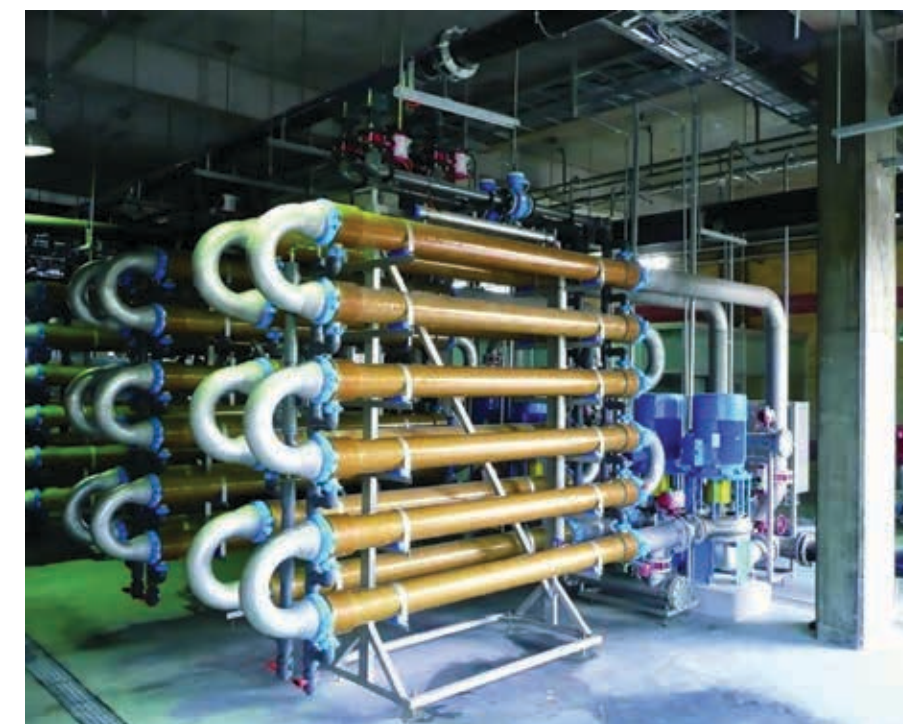
Memthane® combines anaerobic biological wastewater treatment and ultrafiltration in a single process that is ideal for high-strength wastewaters resulting in crystal clear effluents.
