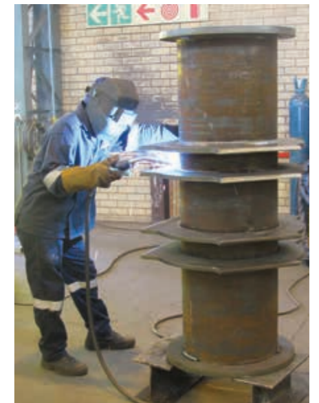
Specialised welding is an integral part of the fabrication and assembly process at Kwatani.
