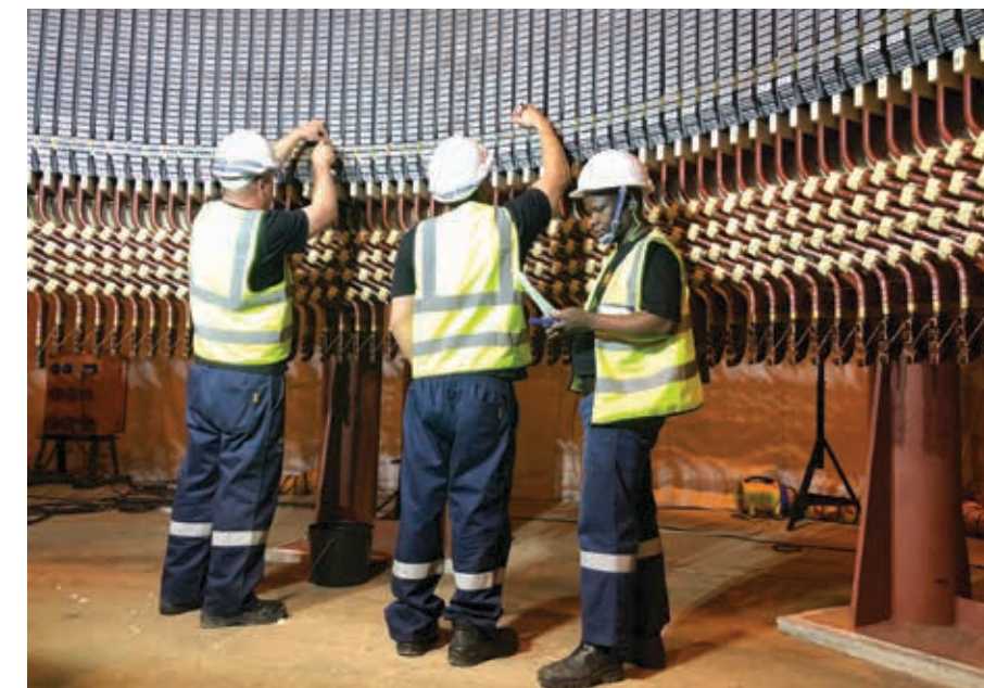
In what has been described as the largest winding installation ever conducted in South Africa, Marthinusen & Coutts has completed a major repair at Eskom's Ingula pumped storage hydro-electric plant. The contract involved the complete rewind of a 373 MVA stator for one of Ingula's four 14-pole motor generators.
