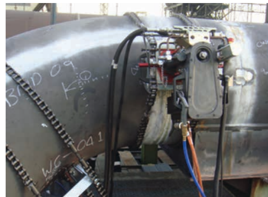
Figure 3: In-situ installation of WeldCore 3 Platform on a steam pipe.
