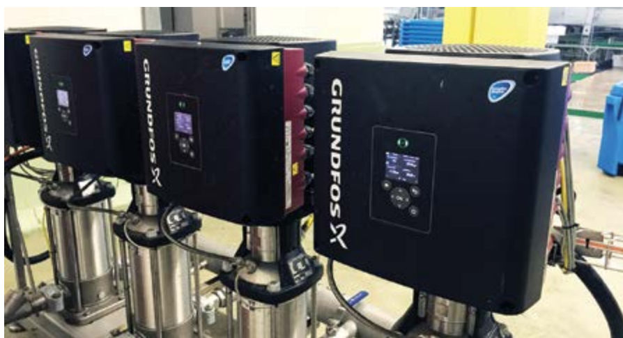
A Grundfos Hydro Multi E booster pump set with HMI display.
