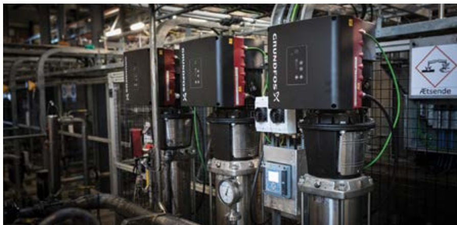
A Grundfos three pump booster set with a cascade function: when flow varies across the plant the booster set can maintain constant pressure with varying flows depending on wash-and-clean demand.
