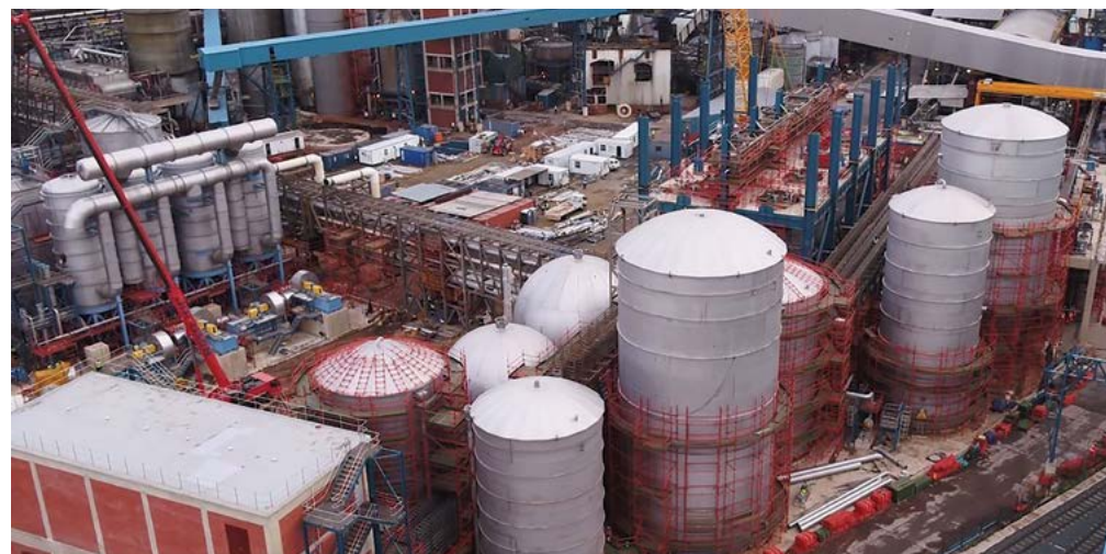
The R7.7-billion Vulindlela expansion project at Sappi Saiccor will increase the mill's production of dissolving woodpulp from 780 000 to 890 000 t/y. Photo courtesy of Sappi.
