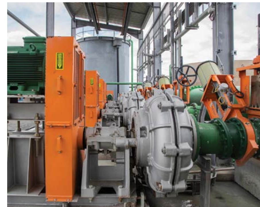
A centrifugal pump driven by a WEG IE4 motor with a VSD can easily result in 15 to 30% energy savings.
