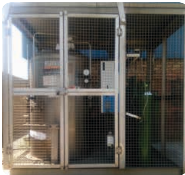
Air Liquide Microbulk incorporates a two or three thousand litre cryogenic argon storage vessel, a CO 2 manifold and Air Liquide's Dynamic Onsite Mixer.
