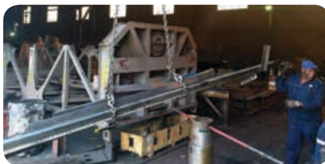
Scheffer Mechanical Technology services over nine mining houses in four groups, which include some of the most globally renowned OEMs.
