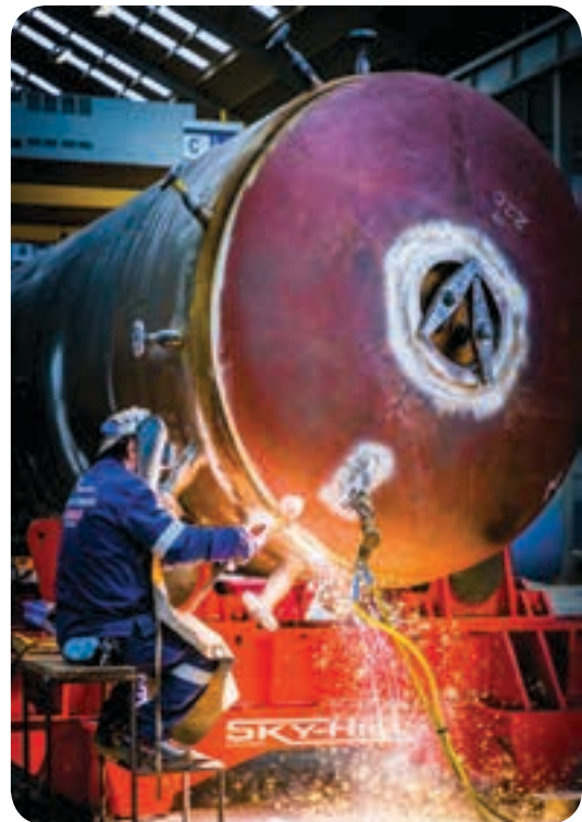
Hydra Arc's state-of-the-art equipment, design capability and skills enable the company to fabricate very large pressure vessels.
