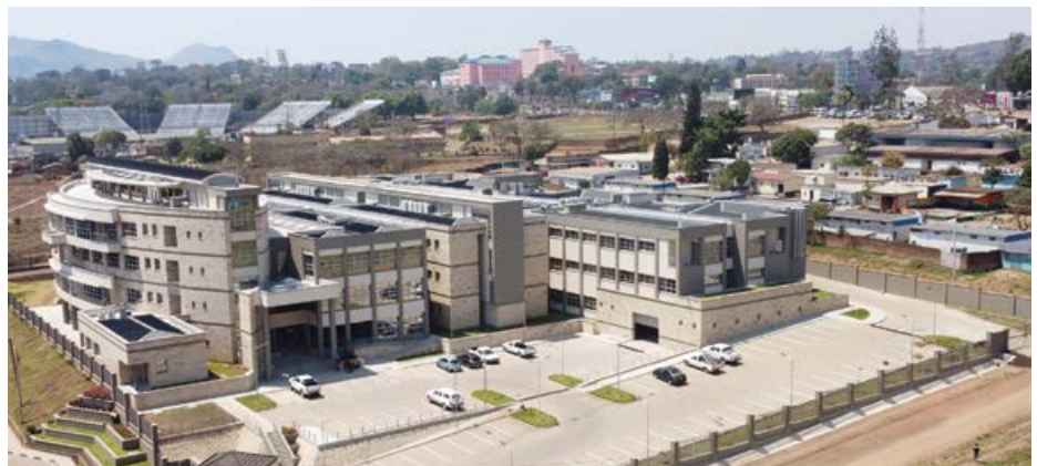
The NDT testing centre will be located within the Malawi Bureau of Standards.
