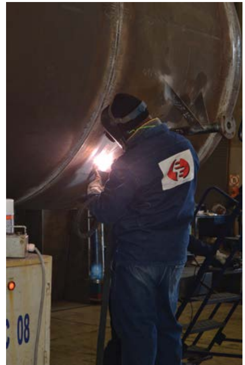
For all welding activities, Efficient Engineering enforces its quality system. "We always have a procedure specification (WPS) that the welders must follow and we call for hold points when inspection must be done," says Dries Vandezande.
