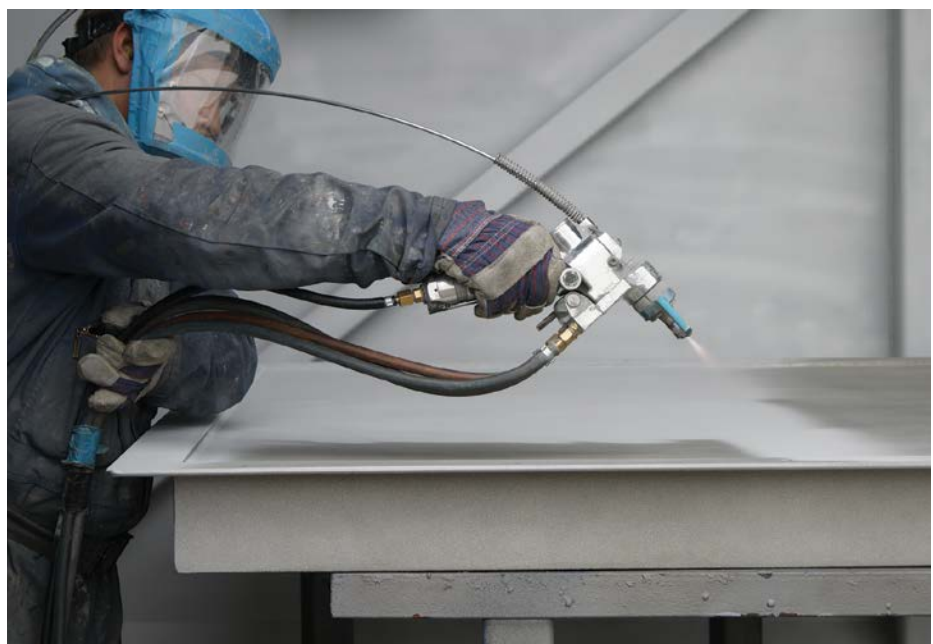
Wire flame spraying of zinc.
