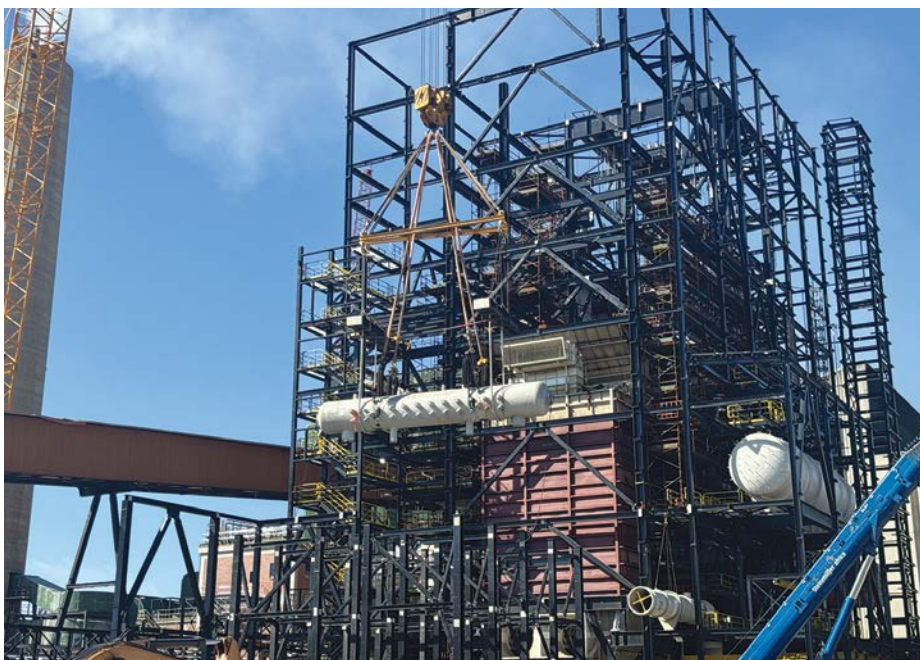
Steinmüller Africa is leading an 18-month boiler construction project for the pulp and paper industry. Shown here is the pre-fabricated steam drum, the heart of the boiler, being lifted into place.
