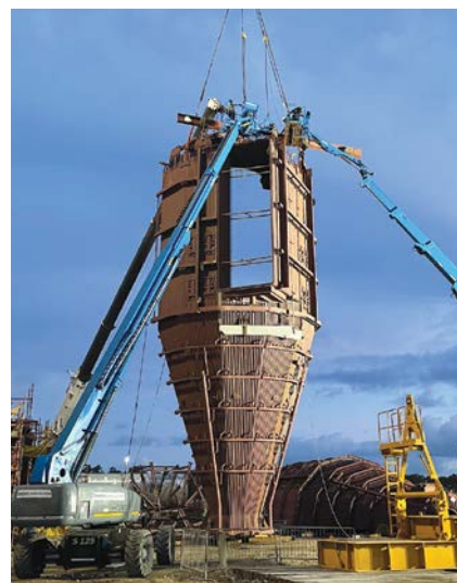
A pre-fabricated conical section being installed in the Mondi boiler.
