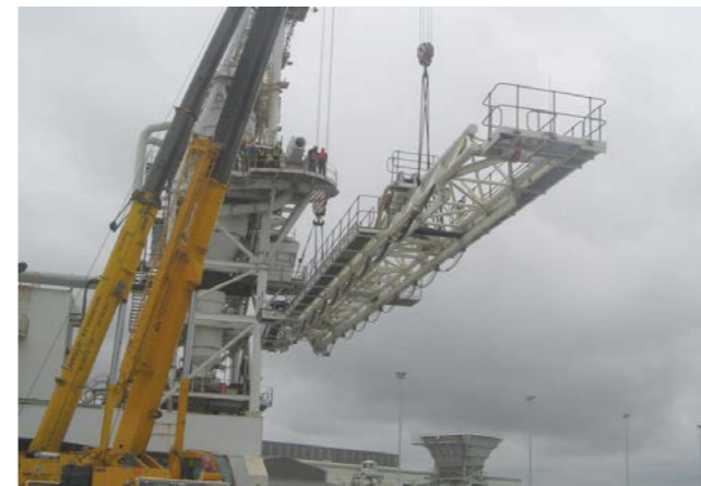
Above: A 42 m boom manufactured and supplied for use on a ship-loader.
