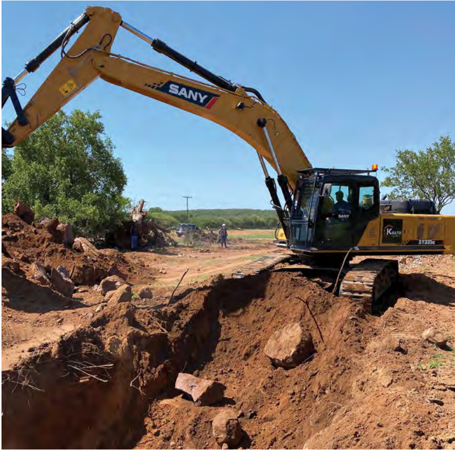
The eight excavators are deployed to lay pipeline sections and backfill material in the trench.
