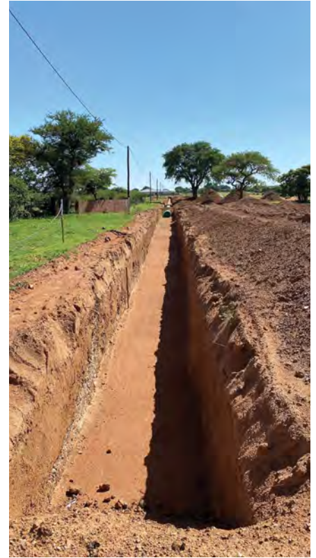
The Masama-Mmamashia pipeline is regarded as a critical piece of infrastructure in the provision of reliable water supply to the heavily distressed southern part of Botswana.
