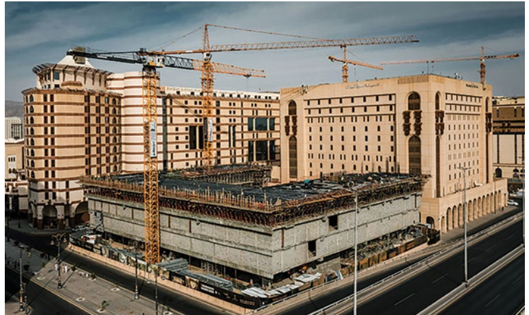
The NC-B 12-70 is suitable for both cast-in-place concrete construction and for the precise lifting of heavy prefabricated parts.
