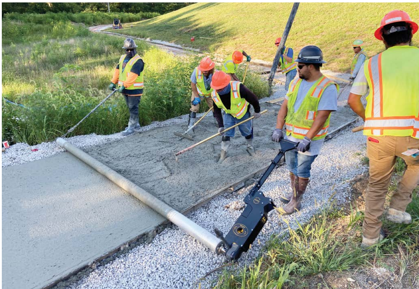
Battery-powered roller screeds provide arguably the most convenient and manoeuvrable screed option available today, with some even providing cross-platform use by utilising the same rechargeable 60-volt lithium-ion battery that is found in common handheld power tools.
