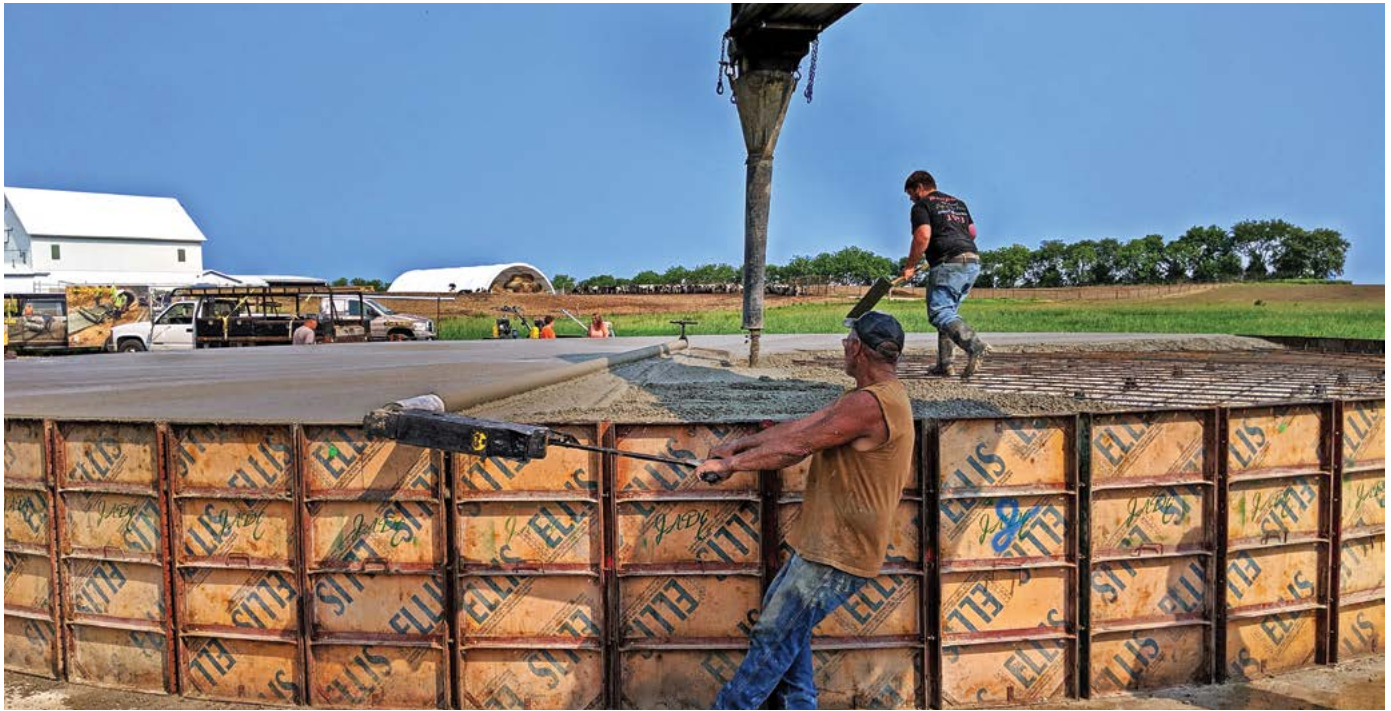
Some screeds, like this one from Curb Roller Manufacturing, provide a single push-button directional change — a convenient feature for special projects, such as circular pours. This allows contractors to easily and quickly change their screeding direction to avoid cold joints and the structural flaws that can occur when concrete cures unevenly.
