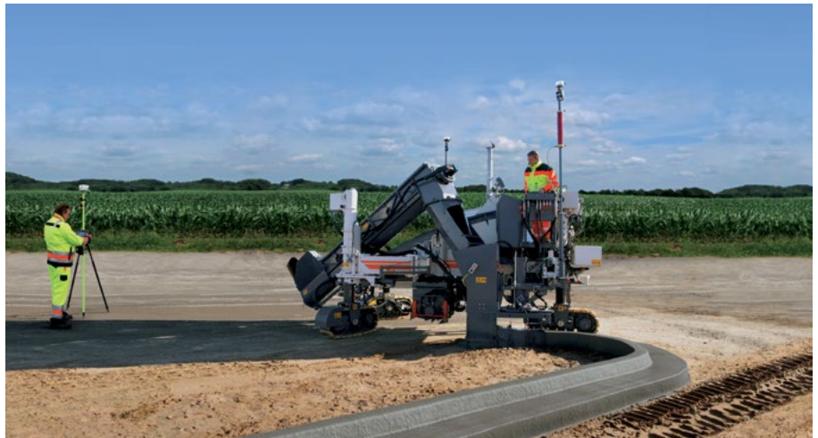
The Wirtgen AutoPilot 2.0 for stringless paving increases process efficiency and safety.
