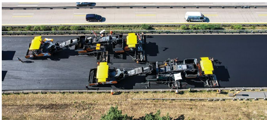
With two InLine-Pave-paving trains from Vögele, the lead contractor rehabilitated a 4.2 km section of the southern part of Berlin's orbital road within two days.
