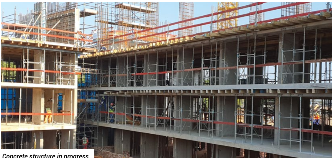
Concrete structure in progress.
