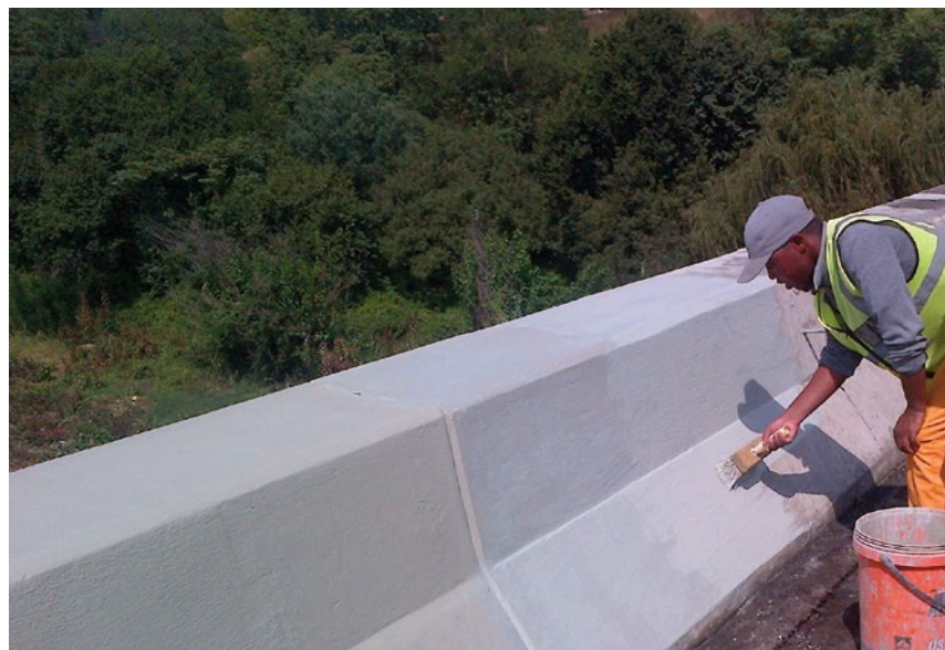
N14 ridges repairs.
