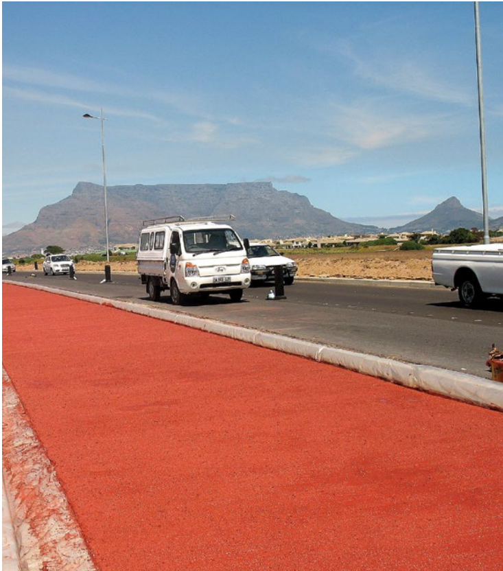
Pigmented concrete bus lanes were innovatively specified for Cape Town's MyCiti public transport system.
