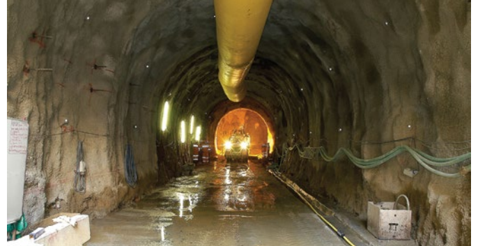
Left: CHRYSO admixtures were used for the incremental launch of the Gilloolys Interchange. Right: CHRYSO Jet accelerators proved invaluable for Gautrain's extensive shotcrete tunnel lining.
