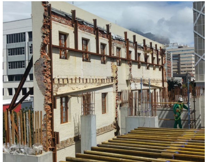
Left: Once completed, the Ikusasa building at the Oxford Parks precinct achieved a 6 star Green Star in terms of the GBCSA Green Star rating. Right: Viewed from inside the 16 on Bree site during construction, the specialised steel bracing used to preserve the 200-year-old façade wall for heritage is visible.
