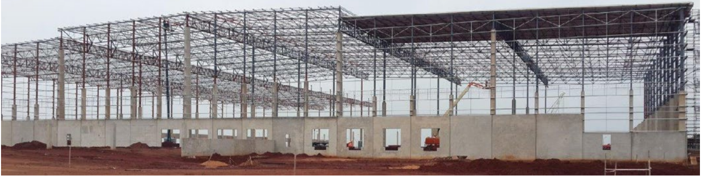
The southern elevation and the five wind-load columns.
