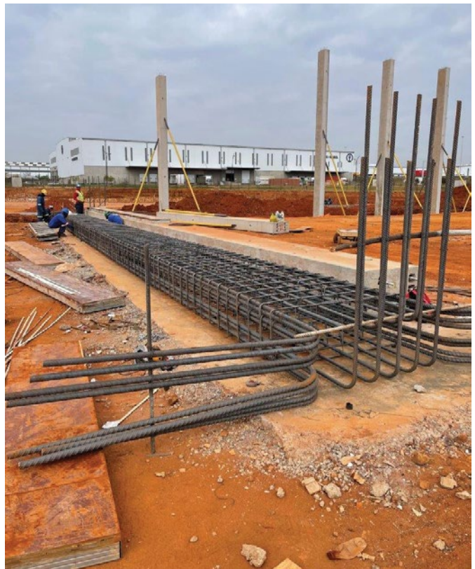
One of the wind-load columns prior to casting.
