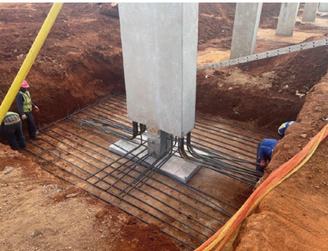
The wind-load columns' starter bars were meshed with the column-base rebar.
