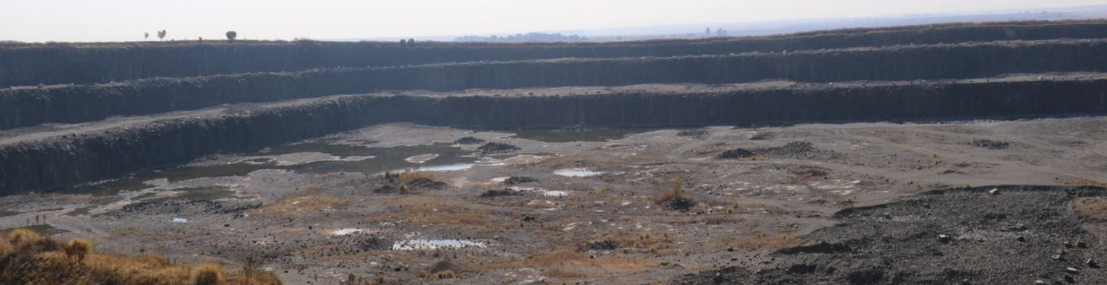
The quarry is a big supplier to asphalt markets which it supplies with its sought-after products – especially 10 and 20 mm road stone.
