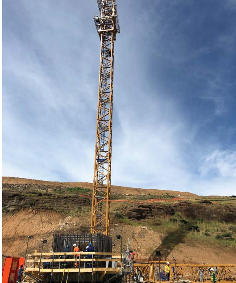
The sliding formwork for Pier 10 (the second highest pier) under assembly. Starting the week of 19 February 2024 and rising slowly and continuously at a rate of 4 m/day the entire 84 m high pier will be cast over 22 days working 24/7 with only one pause at around 60 m, which will be required to extend the tower crane.
