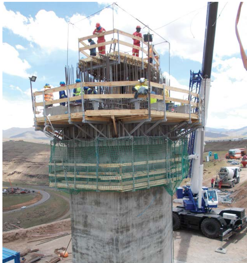
Photo shows how the sliding formwork looks when the contractor slid the first pier (Pier 1) late last year. Top platform is for fixing steel, 2 nd platform for casting concrete and lowest platform for finishing the concrete.
