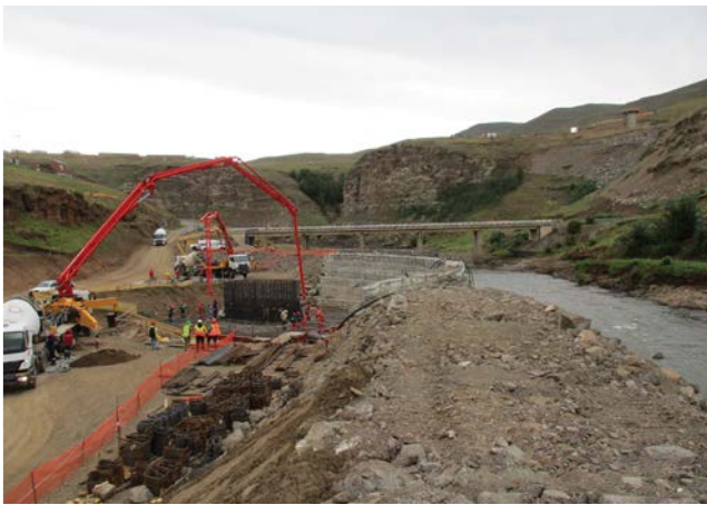
Pier 9 foundation casting. In the background one can see pier 1 which is at the height of the underside of the future deck, Pier 9 will have the highest of the 15 piers reaching approximately 88 m in height.
